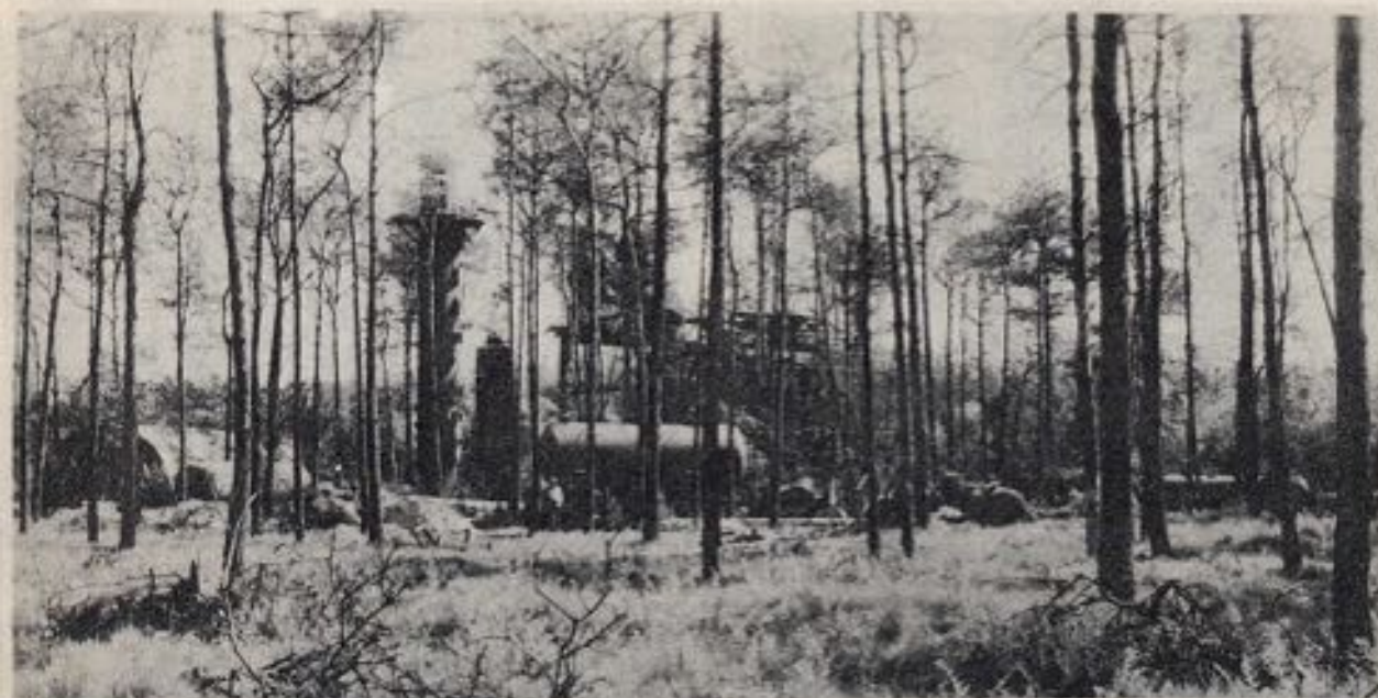
Figure 6 - Little Scholven Hydrogenation Plant - This distillation unit was used with the hydrogenation unit shown on the preceding page. These units were a quarter of a mile apart. The bunker on the left was the control house for this part of the plant.
