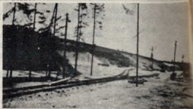
Figure 43 - Concrete Vault at Muehlidorf - The structure is 220 feet wide by 1200 feet long, and the roof is 16 feet thick.
