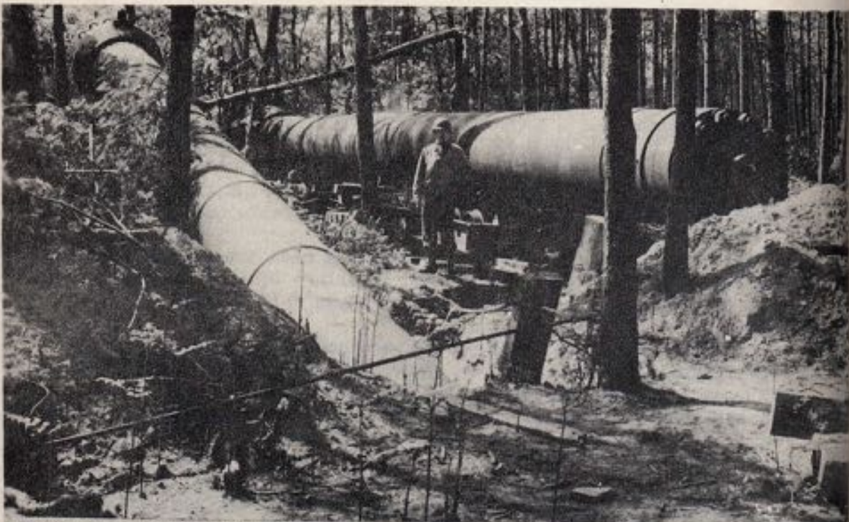
Figure 4 - Little Scholven Hydrogen Plant - After the Scholven plant was bombed, equipment was removed and scattered through a woods near Huels. These ovens are normally vertical but were installed almost horizontally to conceal them despite doubt as to their operability. The one at the left is in operating position.
