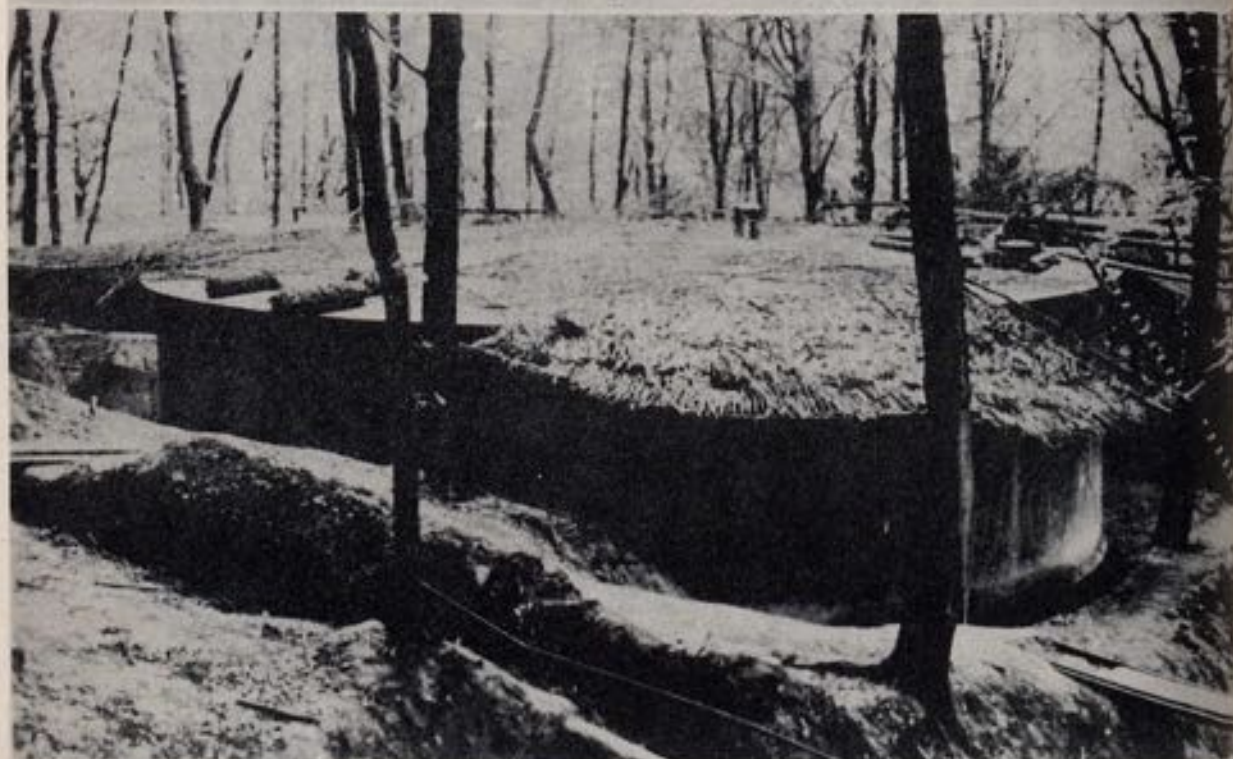
Figure 35 - Underground Lubricating Oil Plant at Porta - The feed tanks were hidden in the woods, but the intermediate storage was underground.
