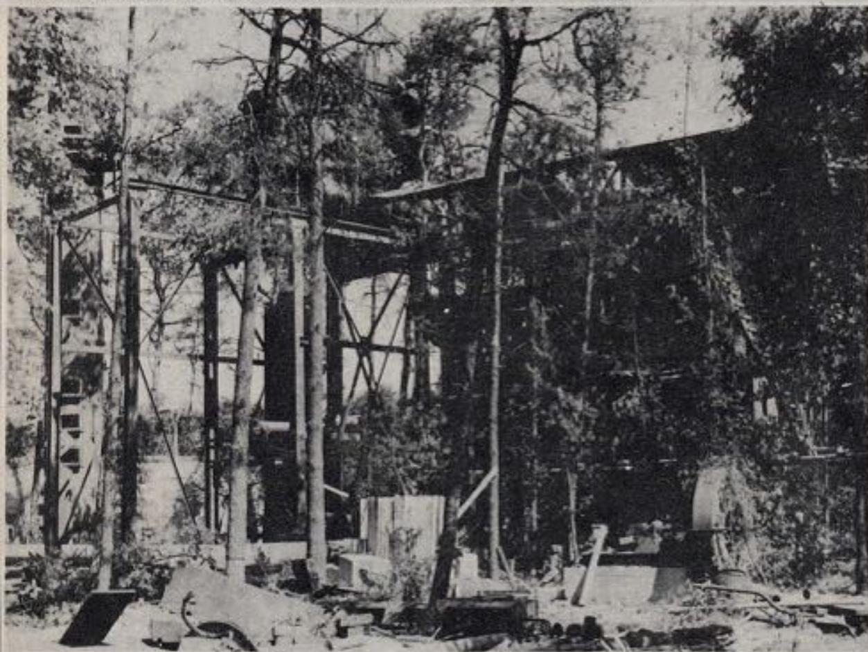
104 Figure 7 - This is a close-up of the distillation furnace and fractionating columns of the plant shown above. This photograph shows the extent to which the equipment was camouflaged: the height of the furnace can be judged by noting the ladder at the right.
