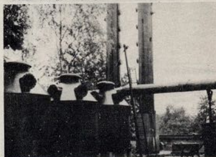
Figure 20 - Fischer-Tropsch Plant at Leipzig - This equipment is used for removing sulphur from the gas fed to the ovens.
