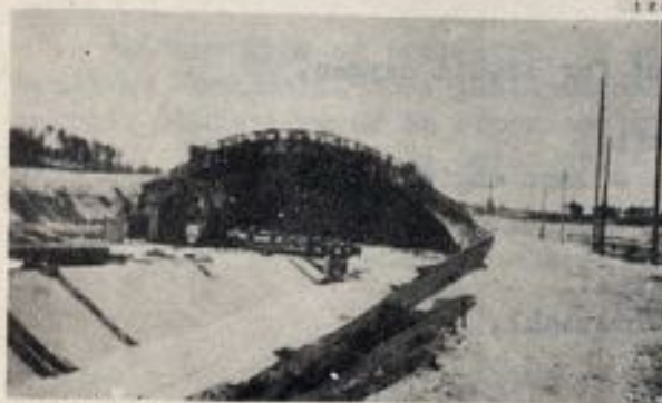
Figure 42 - Concrete Vault at Muehlidorf - Original designed for an eight story airplane factory this shelter was switched to the Buna rubber program. 005
