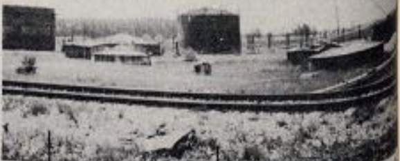
Figure 16 - Cracking Plant at Deggendorf - The tank field was not protected. Dunny tanks were made of plywood and apparently used for quarters.
